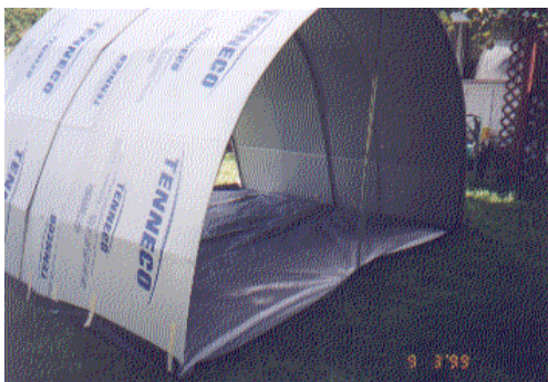
3. Tie fanfold, tape ground film to it.
